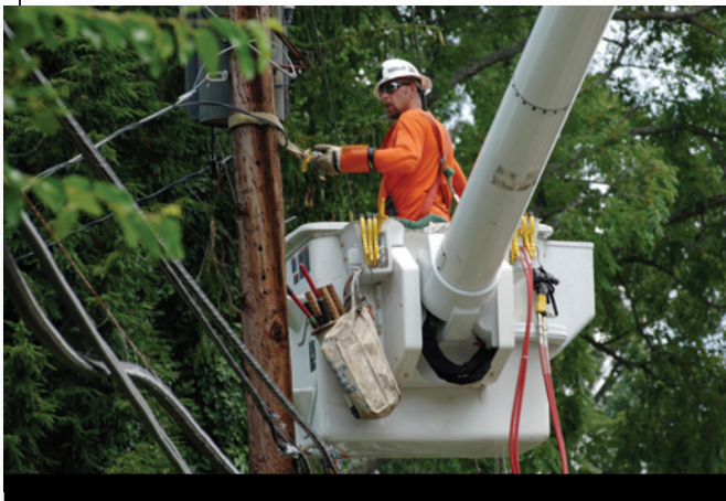
More effective repair crew utilization is the OMS goal.
